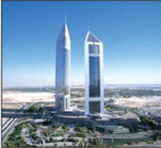
Ssangyong E&C opened doors for other Korean builders to advance into the United Arab Emirates by successfully accomplishing the Emirates Towers Hotel project in Dubai.
